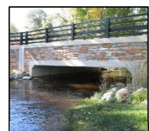
Figure 4: Three-sided box bridge
